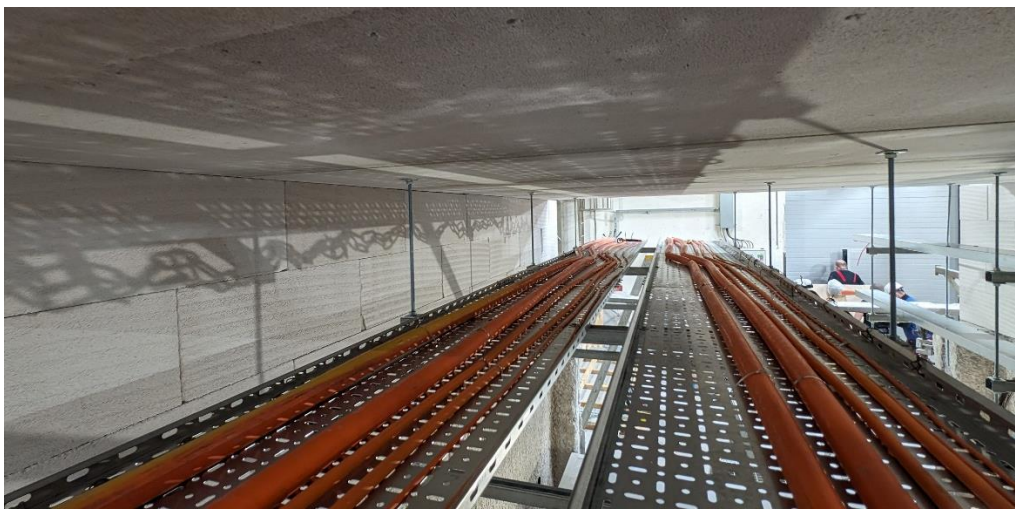
Figure 7 – Armorduct Cable Tray installed in the test furnace.
