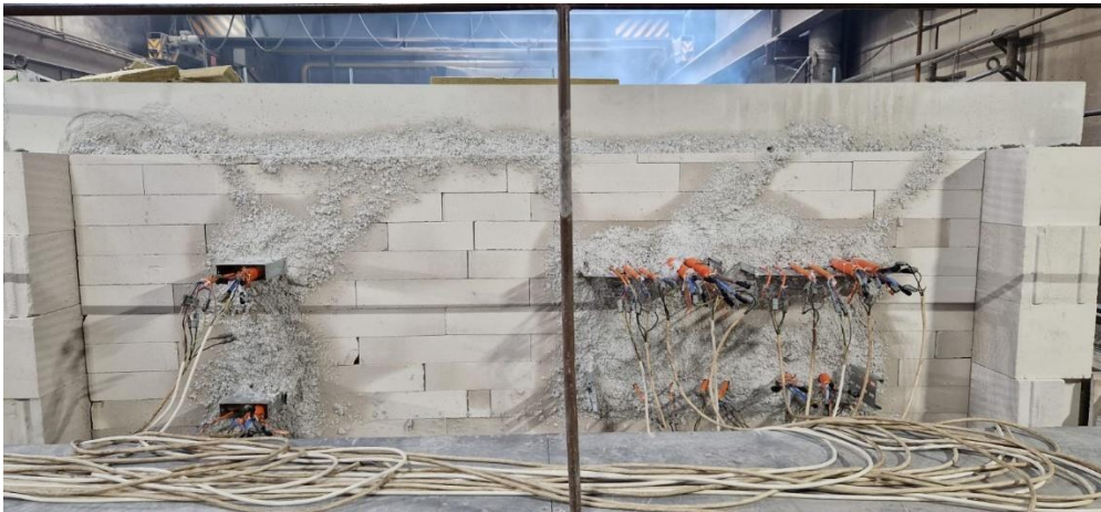
Figure 10 – The completed furnace and cables connected to the current monitoring system.
