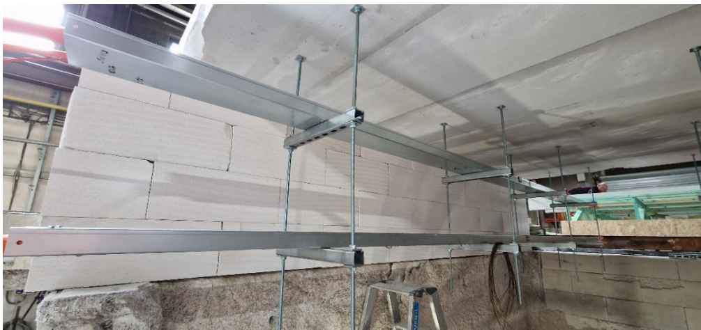
Figure 5 – Armorduct IP4x Cable Trunking installed in the test furnace.
